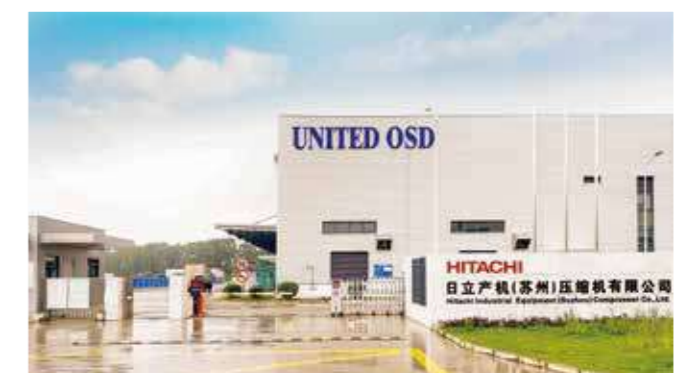
United OSD & Hitachi ISC Joint Production Phase I (Screw & Scroll Compressor)
