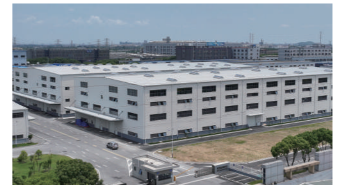
AST Production Plant (Centrifugal Compressor)
