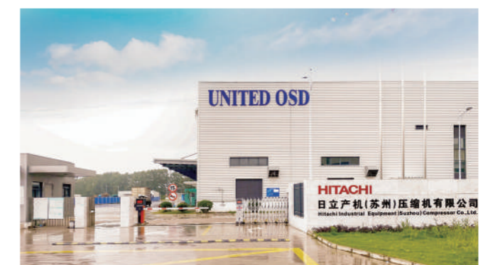
UCS & Hitachi Joint Production Plant (Screw & Scroll Compressor)
