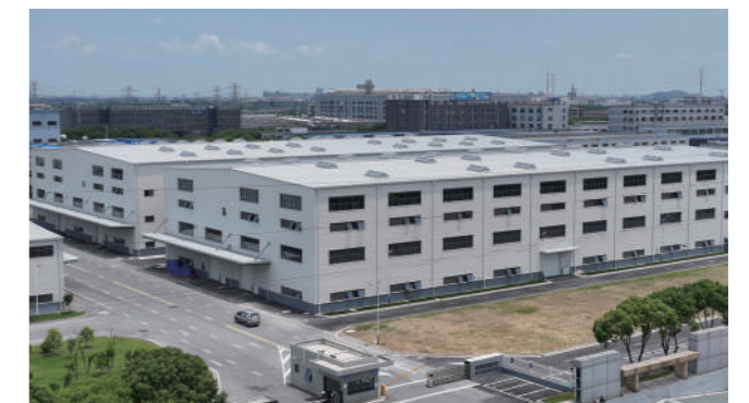
AST Production Plant (Centrifugal Compressor)
