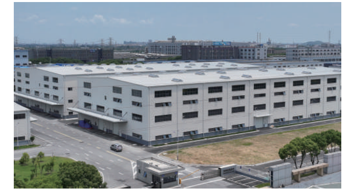
AST Production Plant (Centrifugal Compressor)
